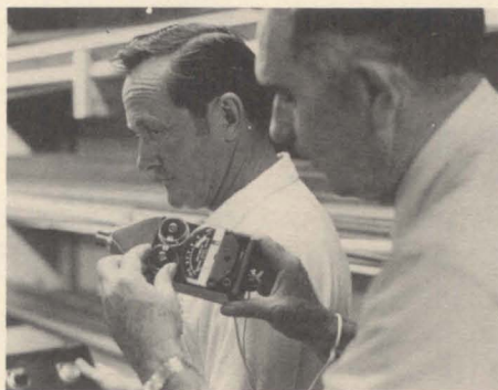
Operating a noise level meter in one of our maintenance locations is Jim Lence , Safety Engineer. Jim holds the meter near Ken Keeb's ear to test the decibel level of noise emitted by a machine he is operating. Ken works in Main Street Maintenance.
